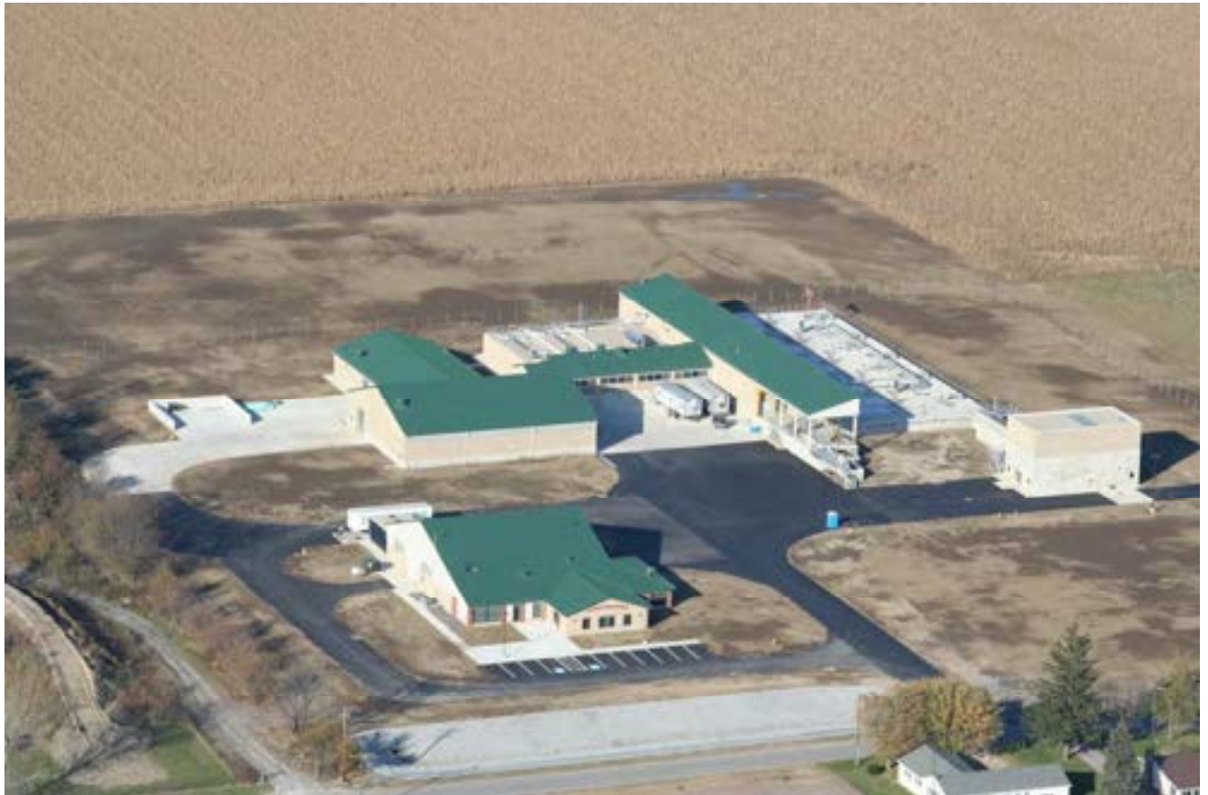
City of Delphos MBR / ThermAer ATAD Wastewater Treatment Facility
