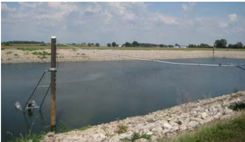
Franklin Storm Lagoon – Increased from 4 to 10 million gallons in 2006
