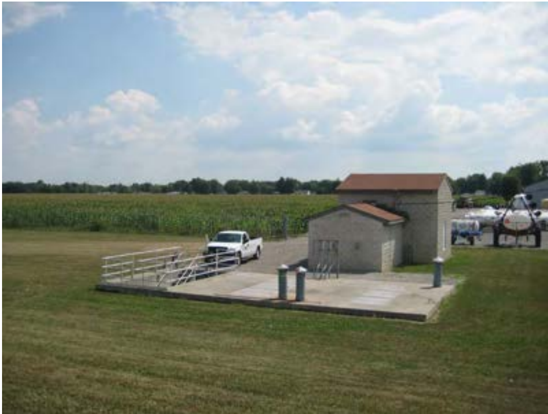
Franklin Street Storm Lagoon Pump Station with bar screen and wet well
